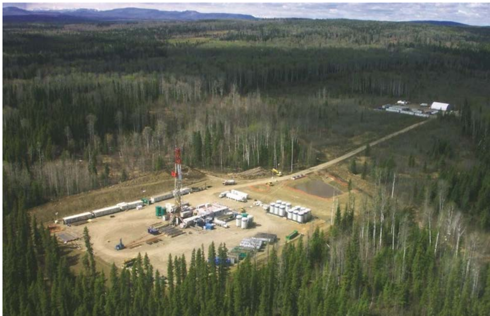
Drilling the exploration well in the Fort Nelson Project area, northeast British Columbia.
